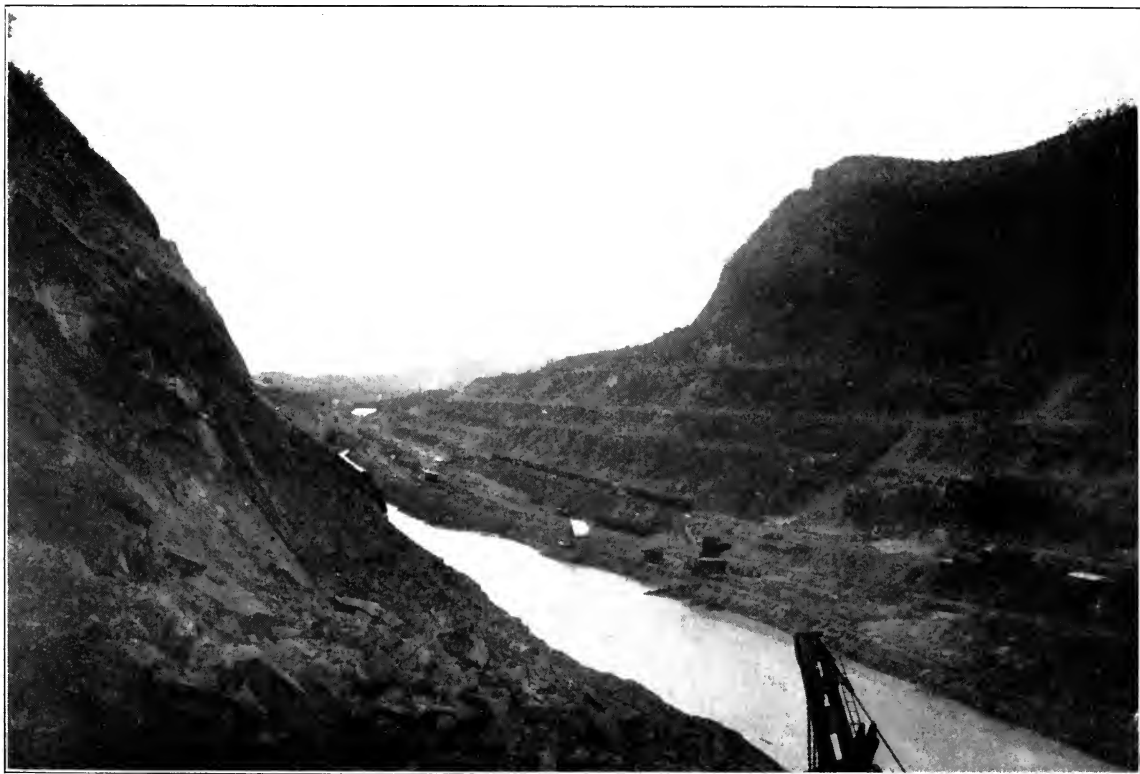
THE CULEBRA CUT, LOOKING NORTH.
